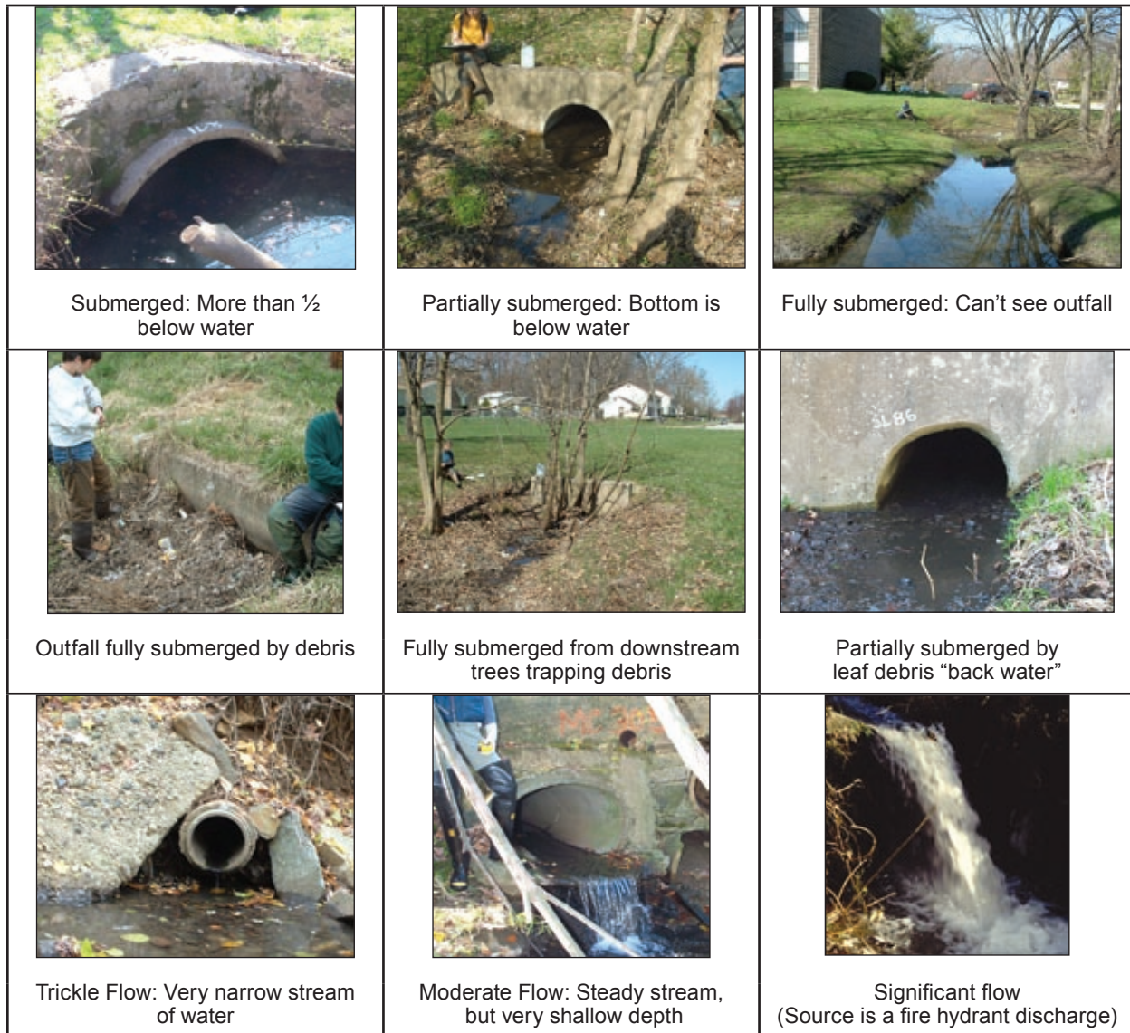
Figure 28: Characterizing Submersion and Flow
