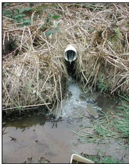
Figure 2: Direct Discharge from a Straight Pipe
