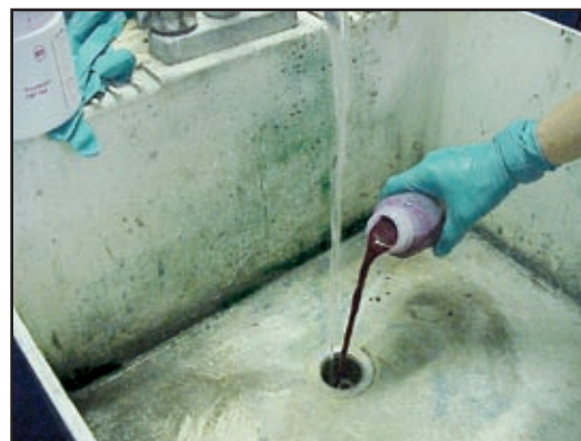
Figure 63: Dye Testing Plumbing (NEIWPCC, 2003)
