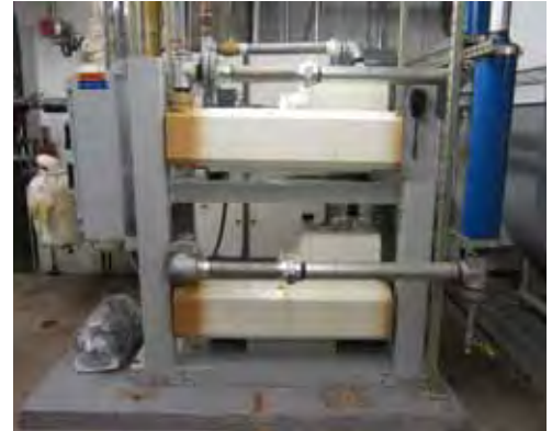
Anesthesia evacuation pumps
