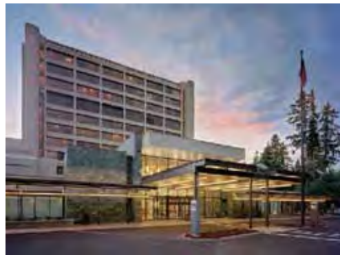
Providence St. Peter Hospital exterior
