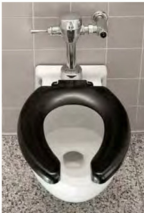
Flushometer-valve toilet
