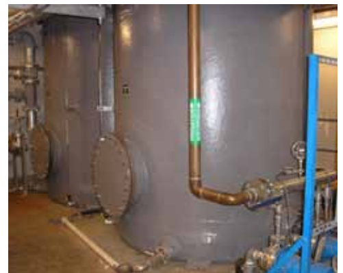
Two 2,500-gallon tanks storing air handler condensate and harvested rainwater for irrigation
